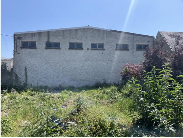
(Above left) External west gable of garage
