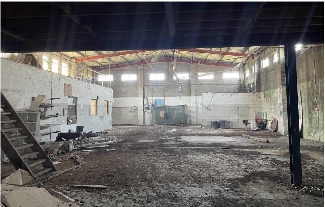
(Below) Garage interior from east
