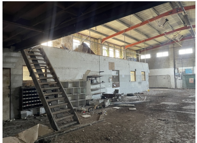
(Above right) Interior view from west of office and main garage space
