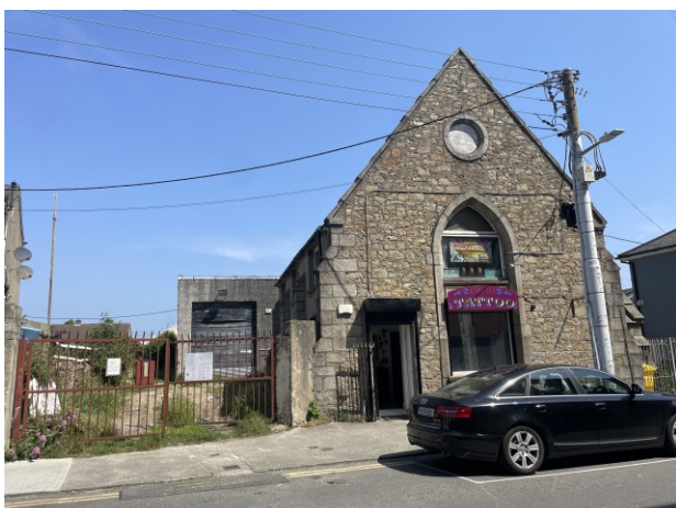
Former Wesleyan Methodist Chapel from Parnell Road now a commercial premises (taken in May 2026)
