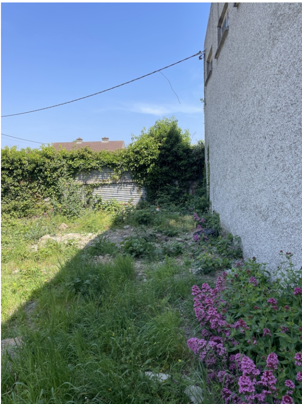
(Below left) Former vehicular entrance in northern boundary wall
